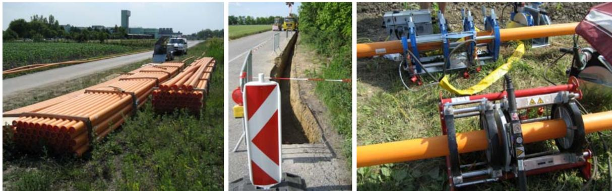
**Figure 10: Biomethane pipeline in Bruck/Leitha, Austria during construction; pipe connection by welding (right); Source: Vienna University of Technology**
